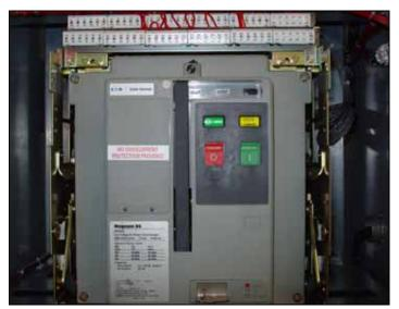
Figure 8. Drawout Switching Device Installed in the Magnum Transfer Switch.
